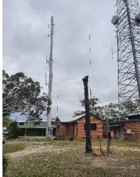
40m concrete monopole
