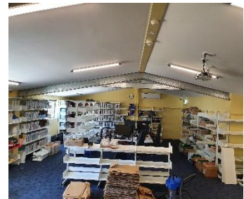
New library extension
