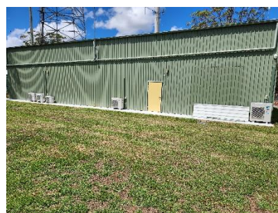
South wall with new exit door.
