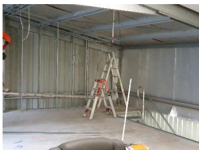
Library extension with new stairs.
