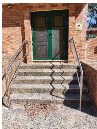
New handrails on VK2WI steps
