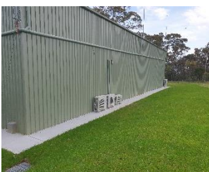
New path on southern side
